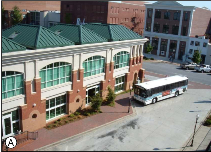
Figure 5.2 Existing Multimodal Center in Spartanburg, SC
