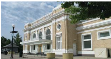
Level 2 Station (Salem, Oregon) Source: WSDOT Archives
