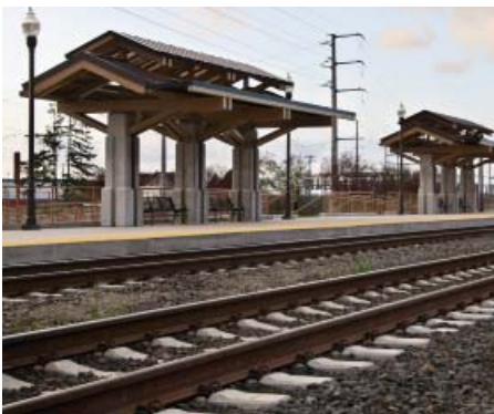
Platform with Partial Canopies at Stanwood Station, Washington Source: WSDOT Archives
