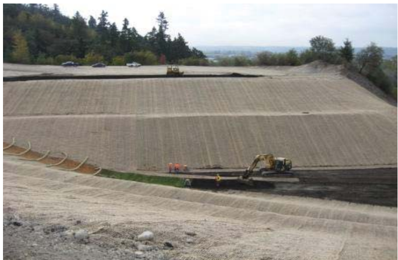
Temporary Erosion and Sediment Control Source: WSDOT Archives
