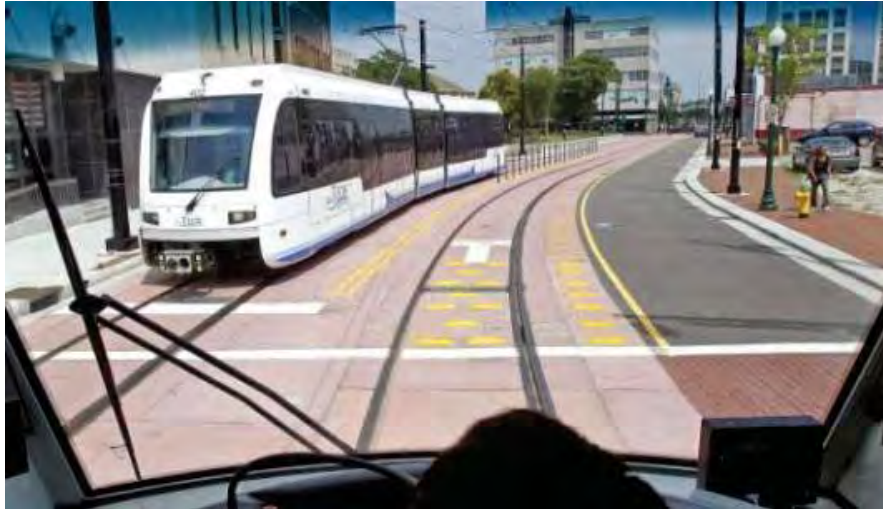
Figure 36 – Plume Street in Norfolk – an example of a Transit Boulevard
