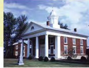
Typical Street view (Stanardsville, Virginia)
