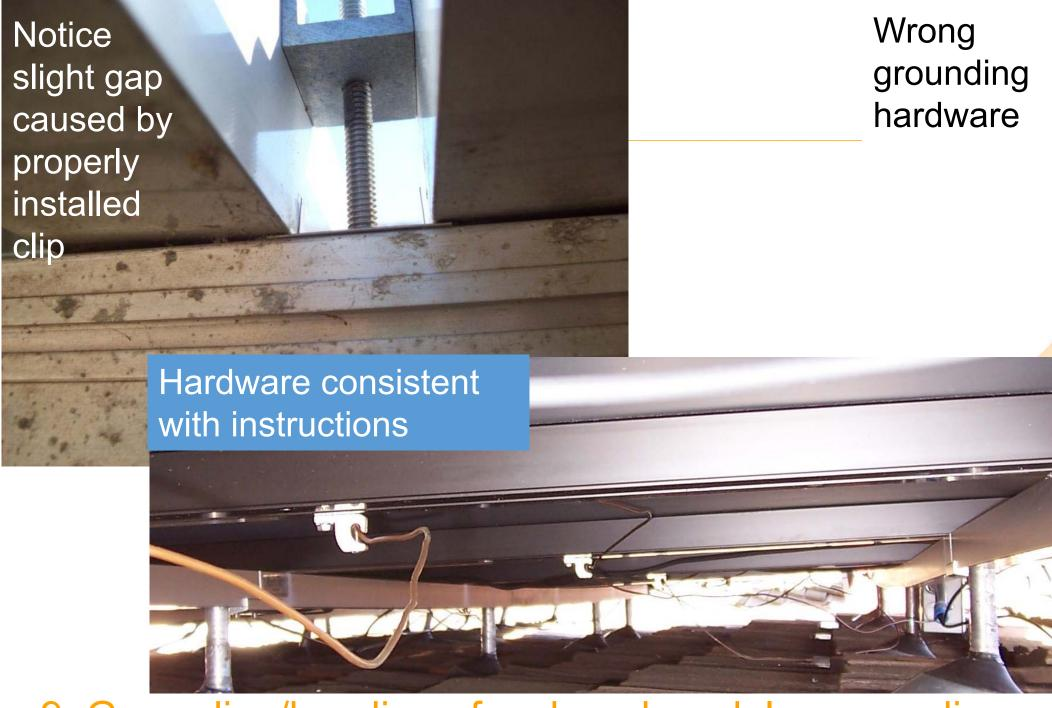
9. Grounding/bonding of rack and modules according to the manufacturer's installation is www.solsmart.org
