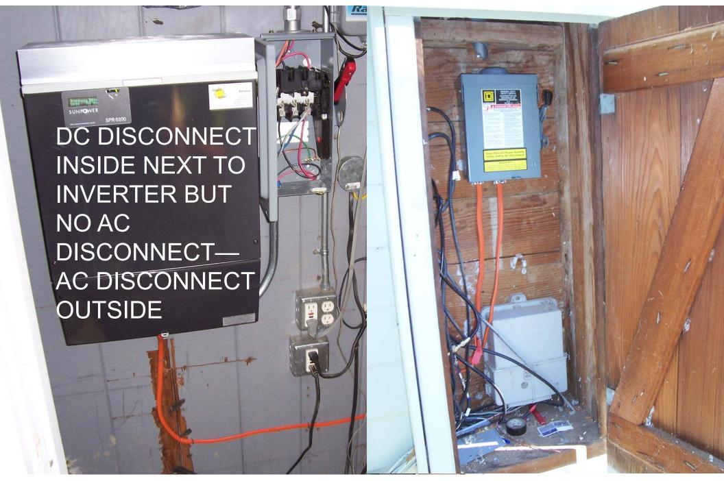
14. Disconnects according to the approved plan and properly located as required to the approved plan
