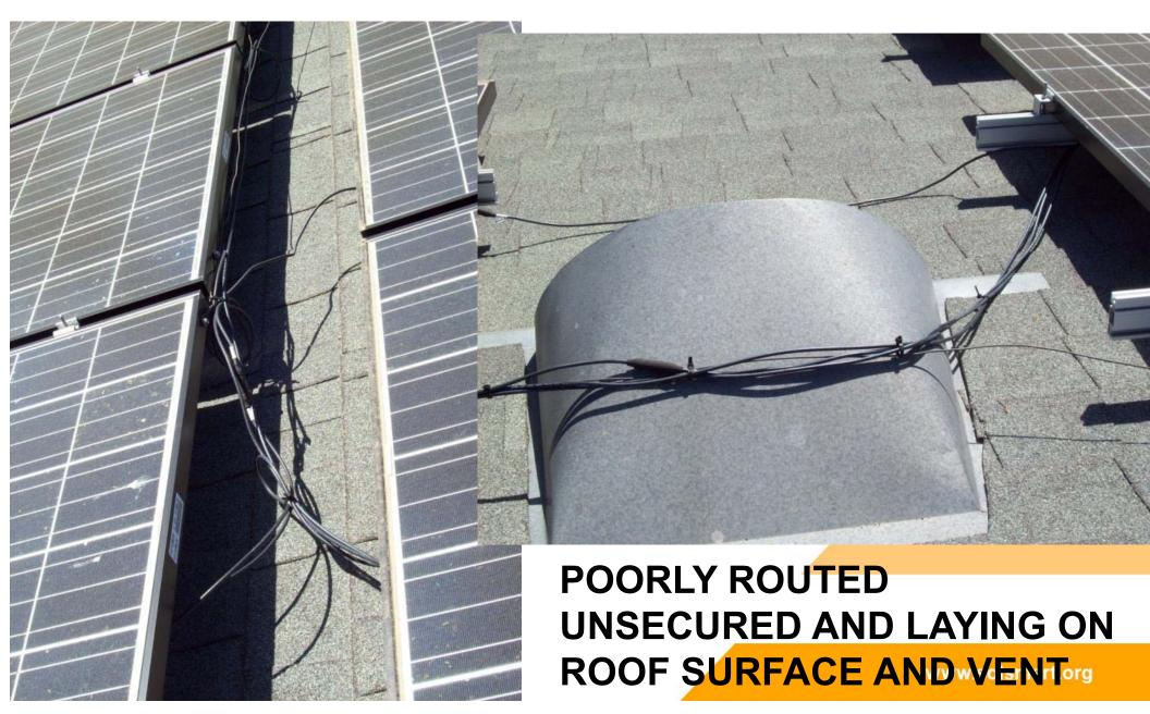
5. Array exposed cables are properly secured, supported and routed to prevent physical damage.
