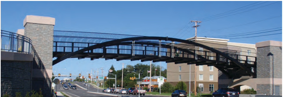
Pedestrian Bridge, Christiansburg
