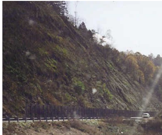
Figure 4.13. Safety fence along I-81 near Christiansburg Mountain
