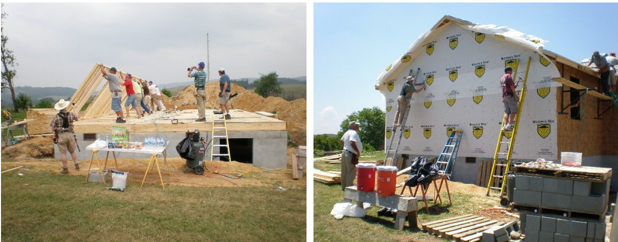
Figure 4.22. Rebuilding Homes Post-tornado in Pulaski County
