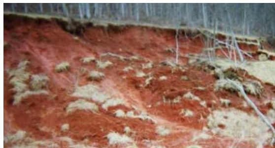
Figure 4.8. Minor landslide in Elliston, February 2003
