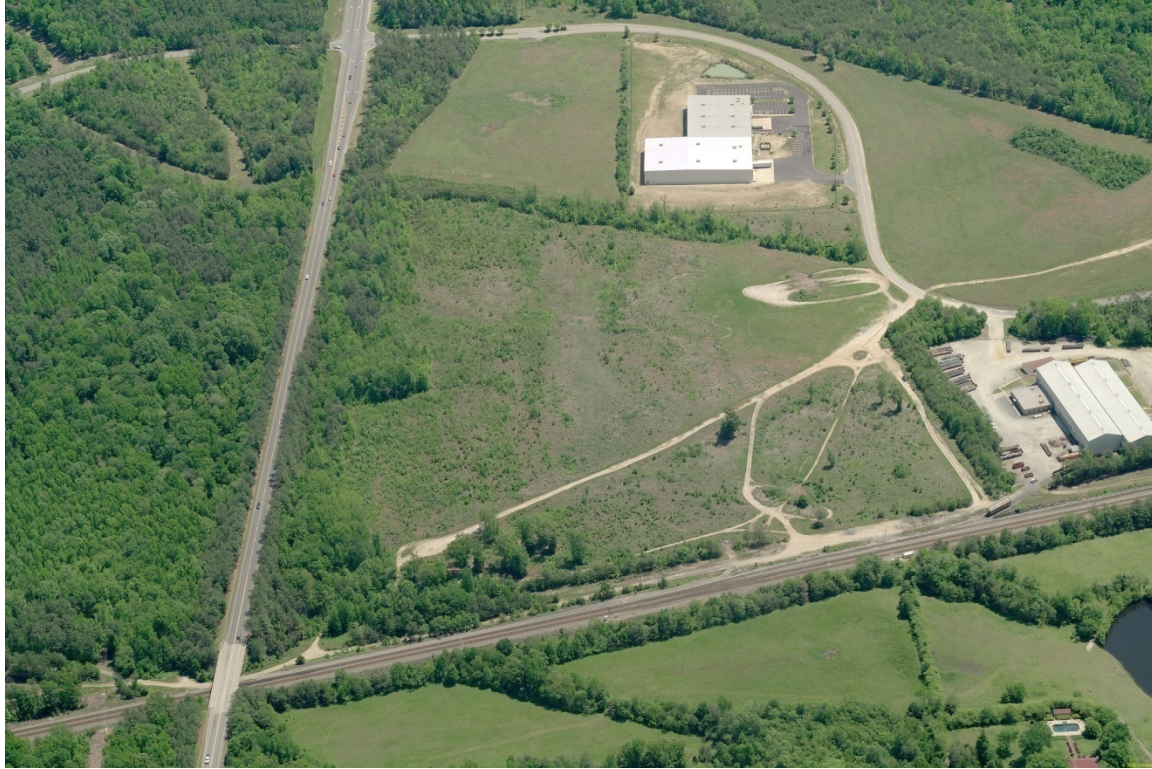
1: Site 1A Facing East
