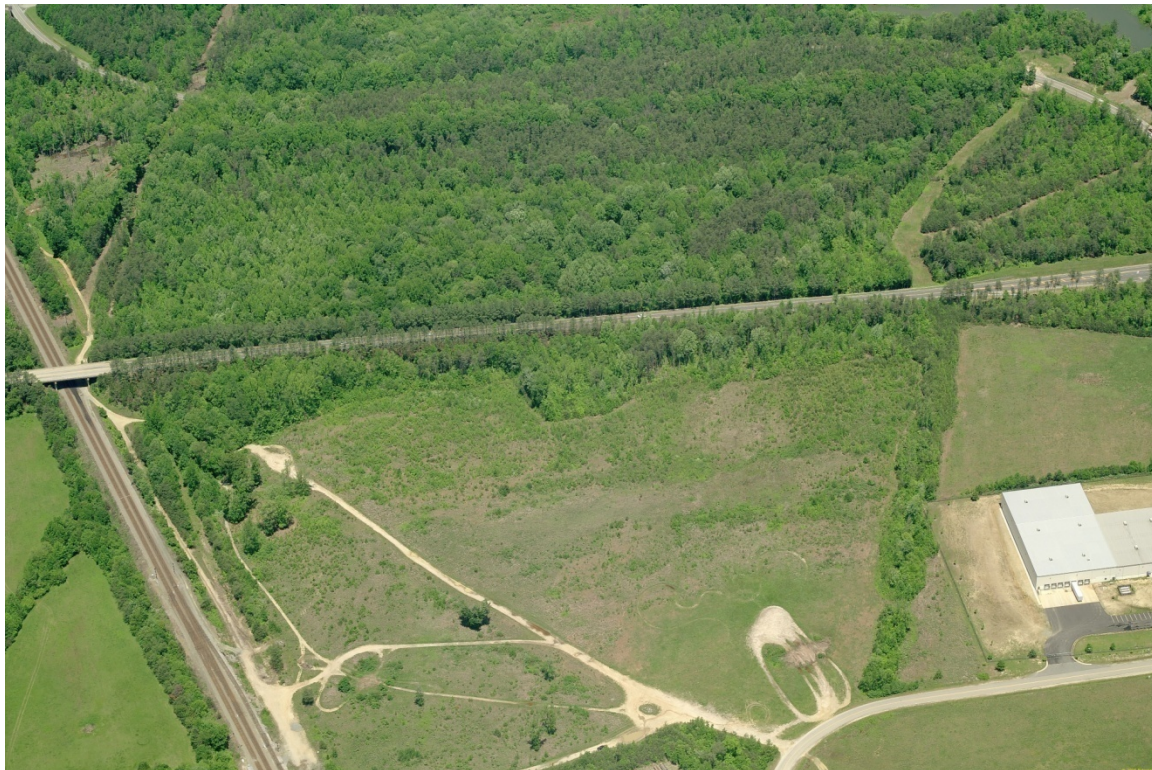
2: Site 1A Facing North
