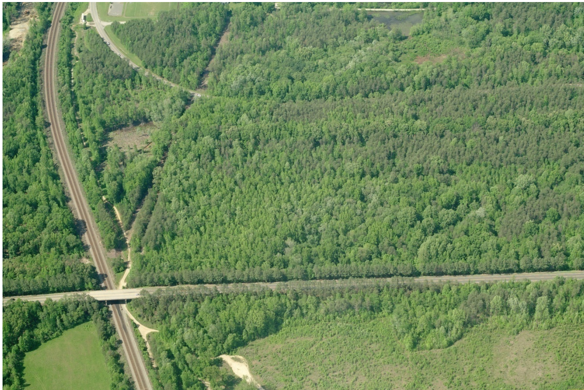
4: Site 2A Facing North
