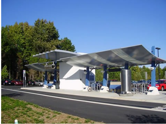
This PNR separates auto, bus, and pedestrian traffic, and provides comfort, security, and convenience to passengers
