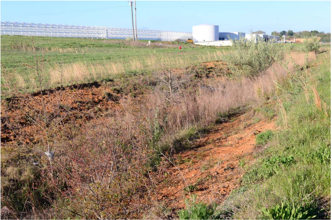
Roadside swales unmaintained
