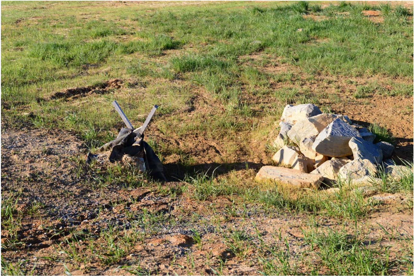
Old temporary ENS measures were never removed
