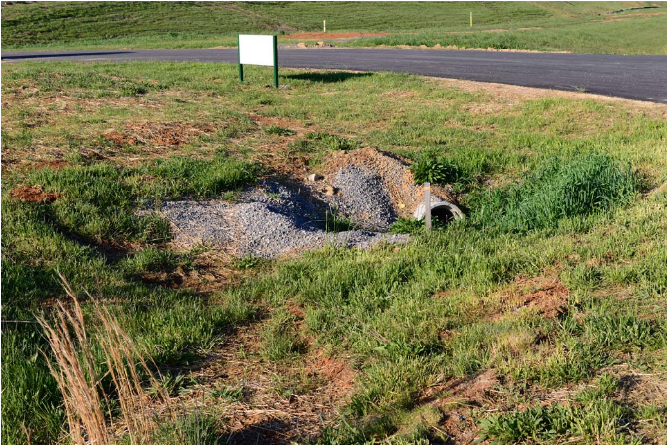
Old temporary ENS measures were never removed
