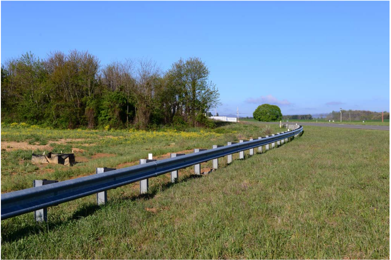
Guard rail no longer needed- to be removed
