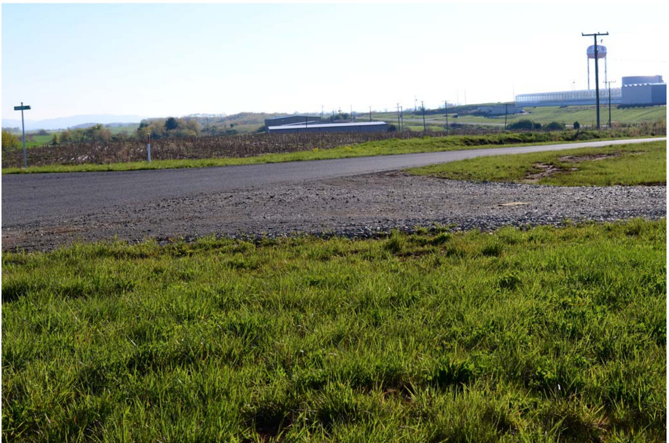
Missing culvert under entrance
