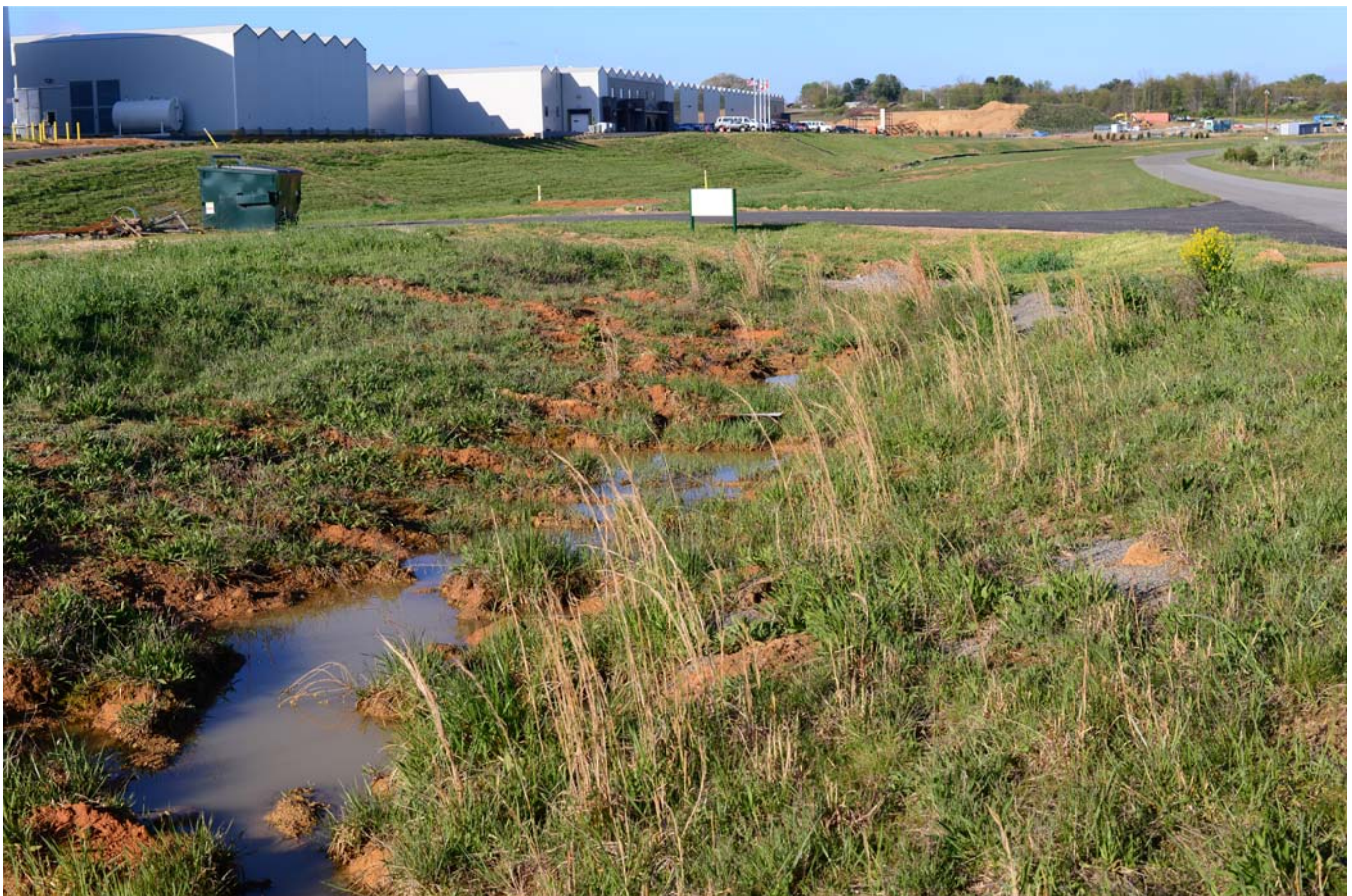
Lack of positive drainage in swales
