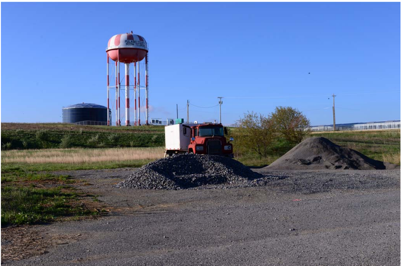
No turnaround at end of road
