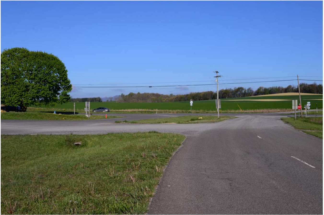
Intersection spacing and culvert
