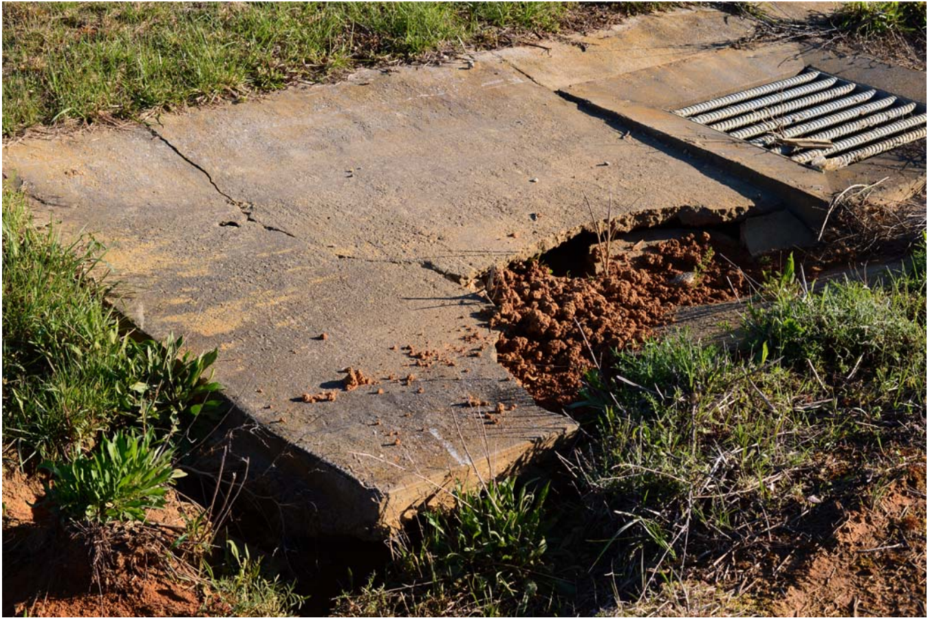
Broken drainage structure
