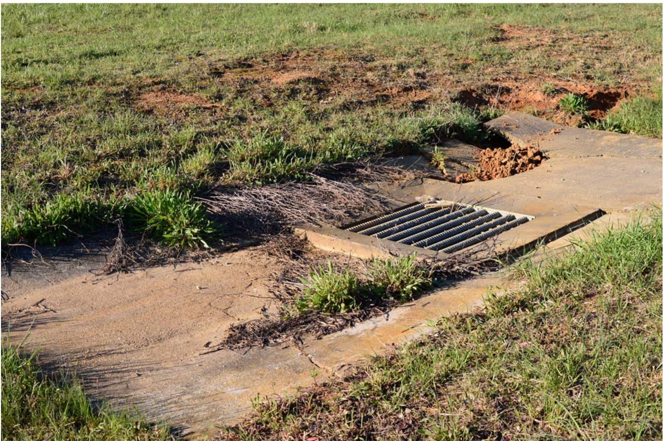
Broken drainage structure
