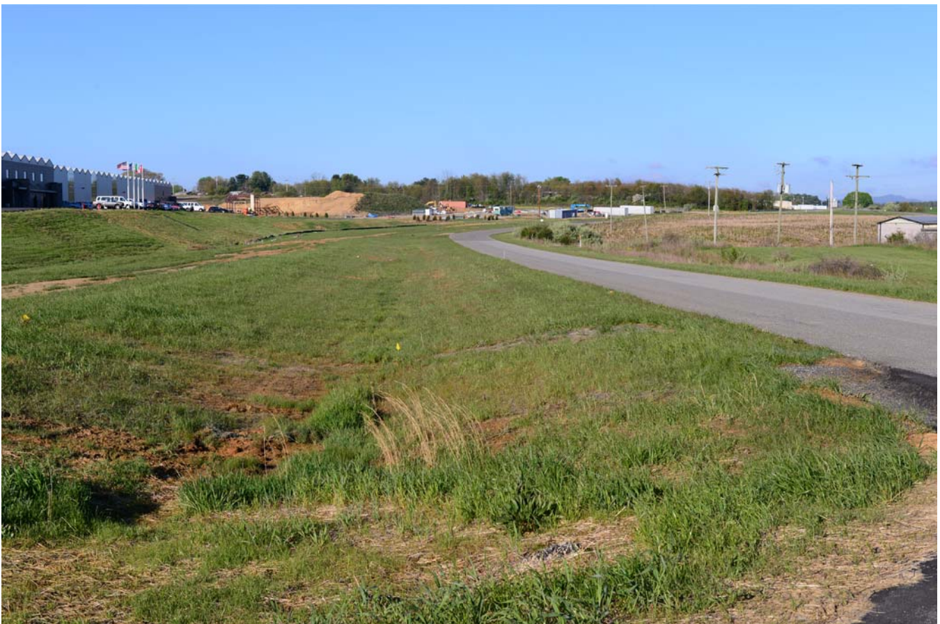
Lack of positive drainage in swales
