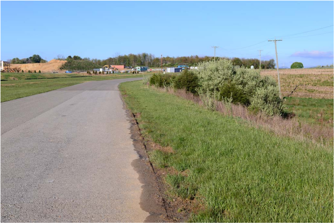
Lack of swale/ soft shoulders
